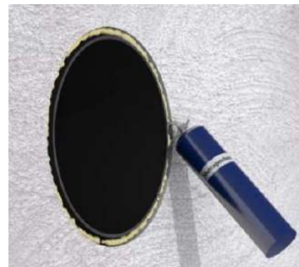
Fig. 5 Sealing the wall mounting pipe
