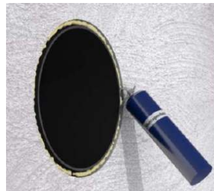
Fig. 5 Sealing the wall mounting pipe
